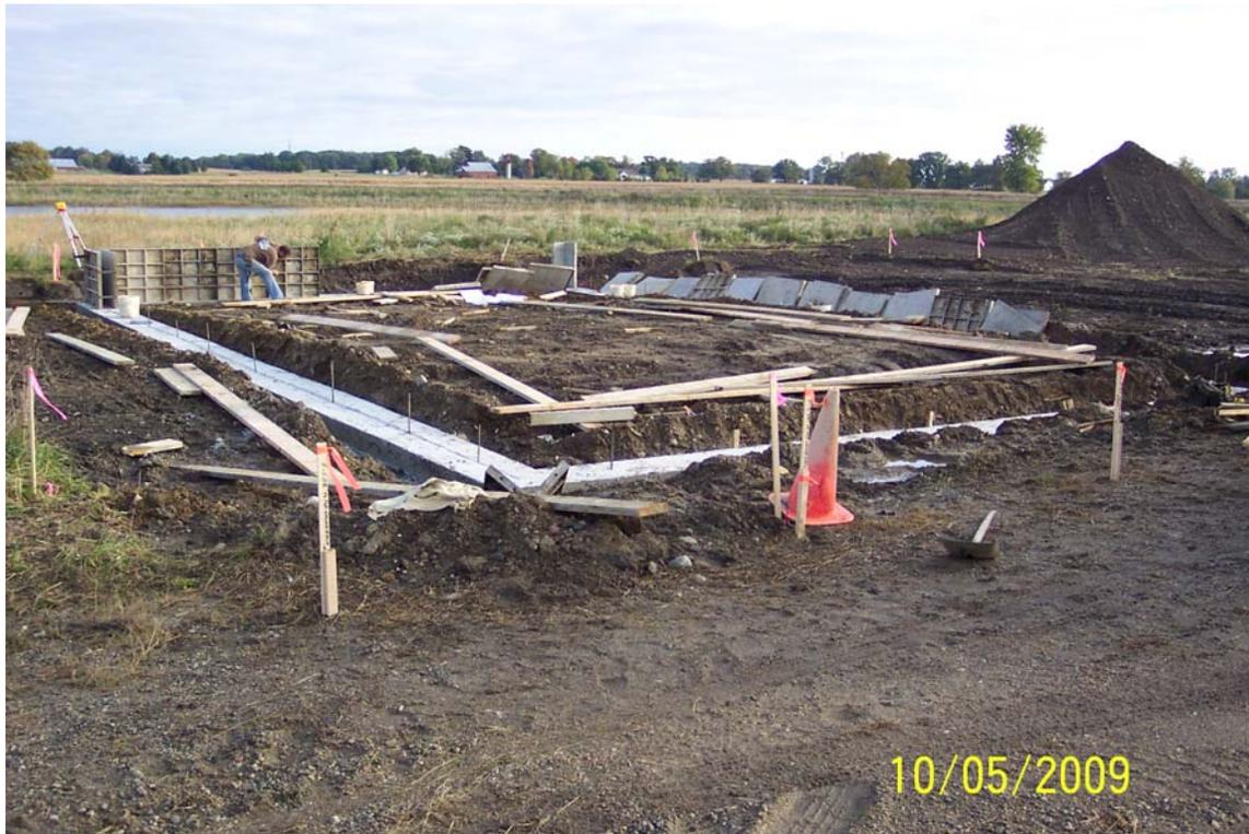
**Top:** Foundation forms are being positioned on top of concrete footings. Once poured the footings/foundation will support the weight of the Beach House's block walls.
