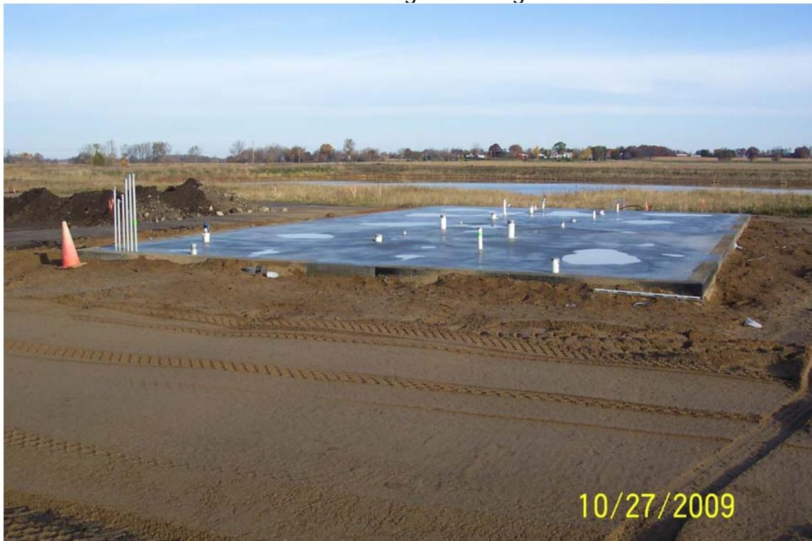
By the time the Green Space Commission meets on November 2, the contractor will have installed the group pavilion's post piers and concrete floor. The pedestrian walkway that fronts on the vehicle parking area will also be completed. The walkway is needed to establish an elevation reference point from which to construct the base for the parking area. All the remaining concrete flatwork and asphalt surfacing of the entrance drive and parking lot will be put off until next spring.
