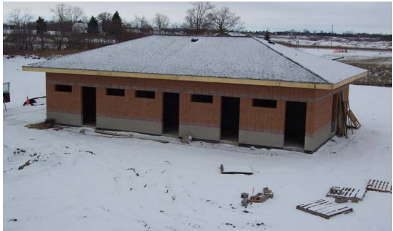
Motz County Park beach house construction progress photo taken 12/23/09.
