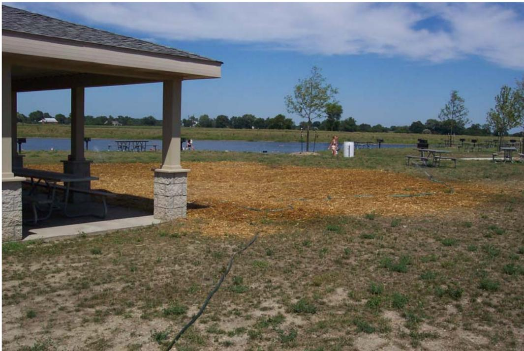
In late July, Cross Lake Construction contoured the ground east of the pavilion to enhance surface water flow towards an existing underground drain. This work was completed to eliminate floor flooding that was occurring at the east end of the pavilion.
