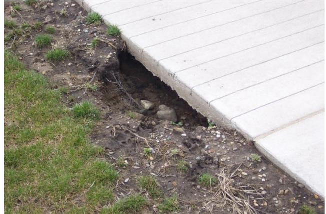
Ground erosion up-slope from the sun beach allowed surface water to flow under the walk for a distance of 85' to 100' resulting in removal of supporting sand.
