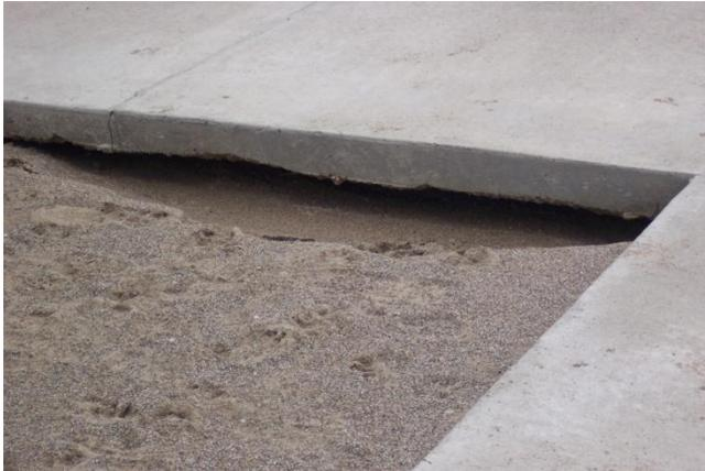
Shown is one of several areas where recent rains resulted in almost complete loss of sub-base under the main pedestrian walk to the beach. Photo taken: April 23, 2013
