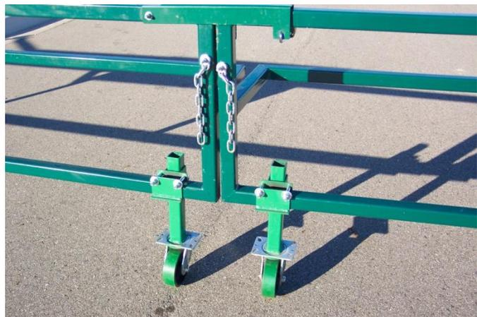
Wheels added to park entrance gate to support the weight of the gate arms and align the two arms for locking.
